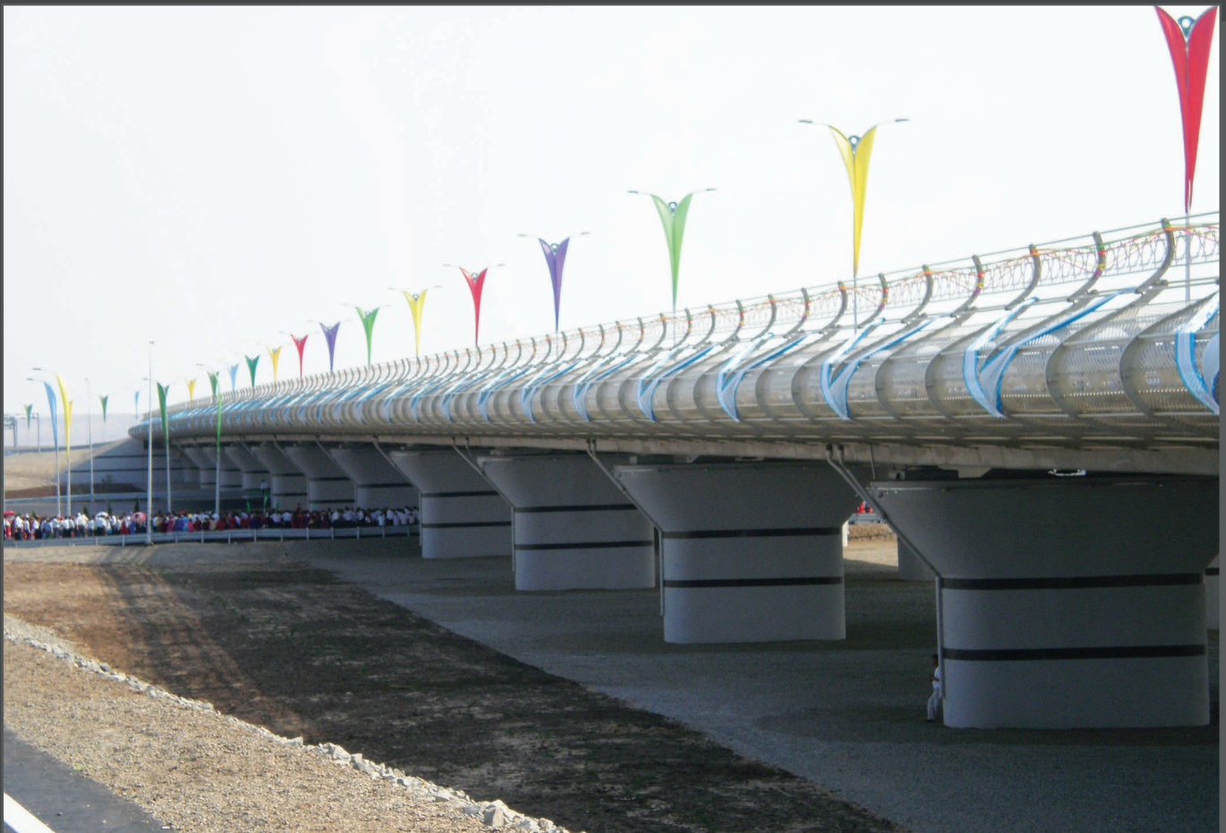
• TURKMENISTAN - Avaza Bridge
